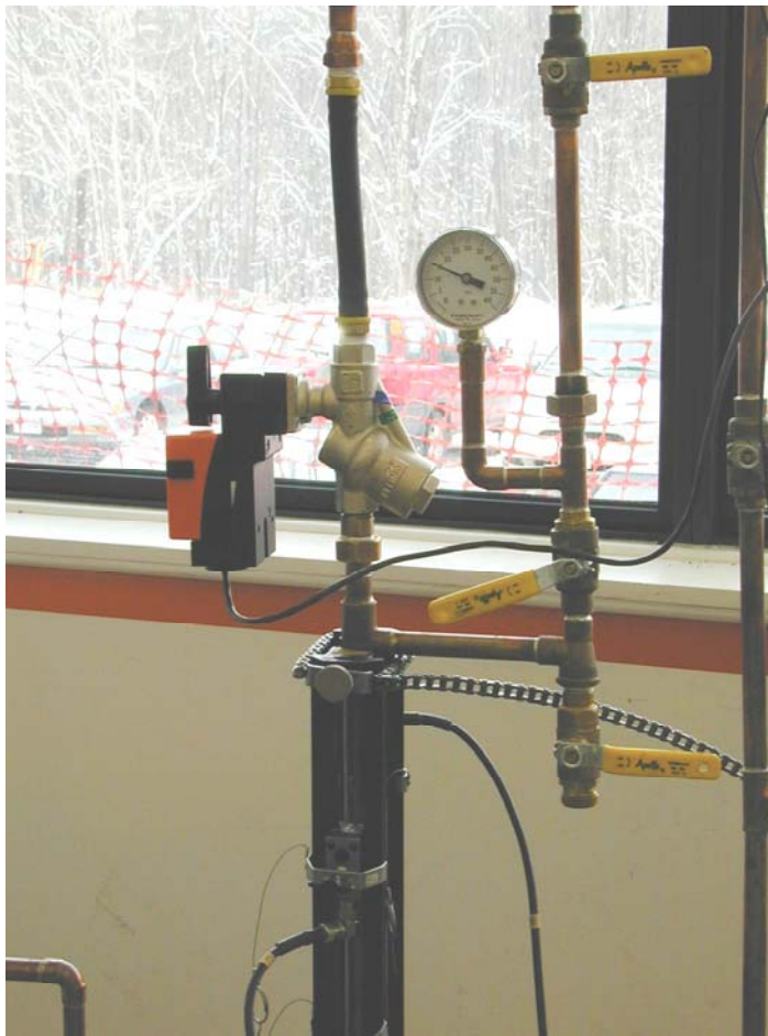
Plate 4 ½ inch valve under test
