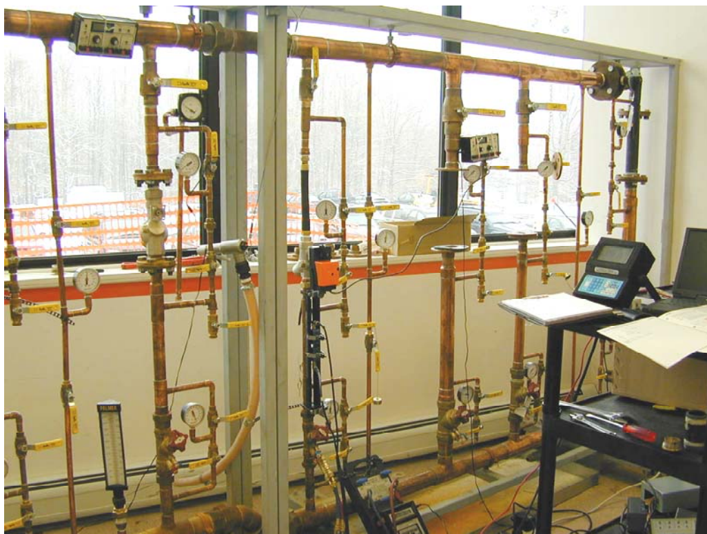
Plate 3 General view of PICCV test rig
