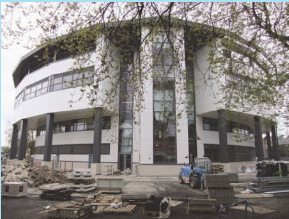
Airtightness testing at an academy in Hammersmith
