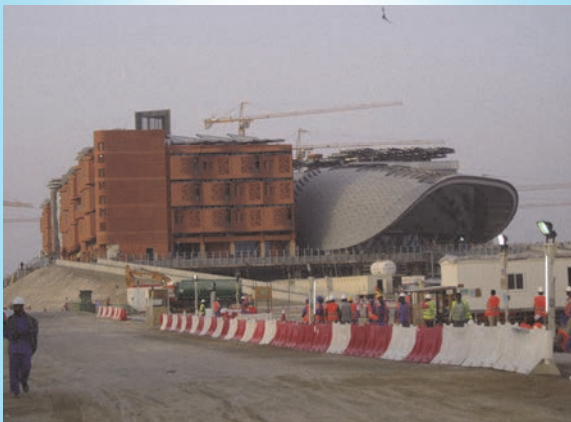
Airtightness testing at an academy in Abu Dhabi
